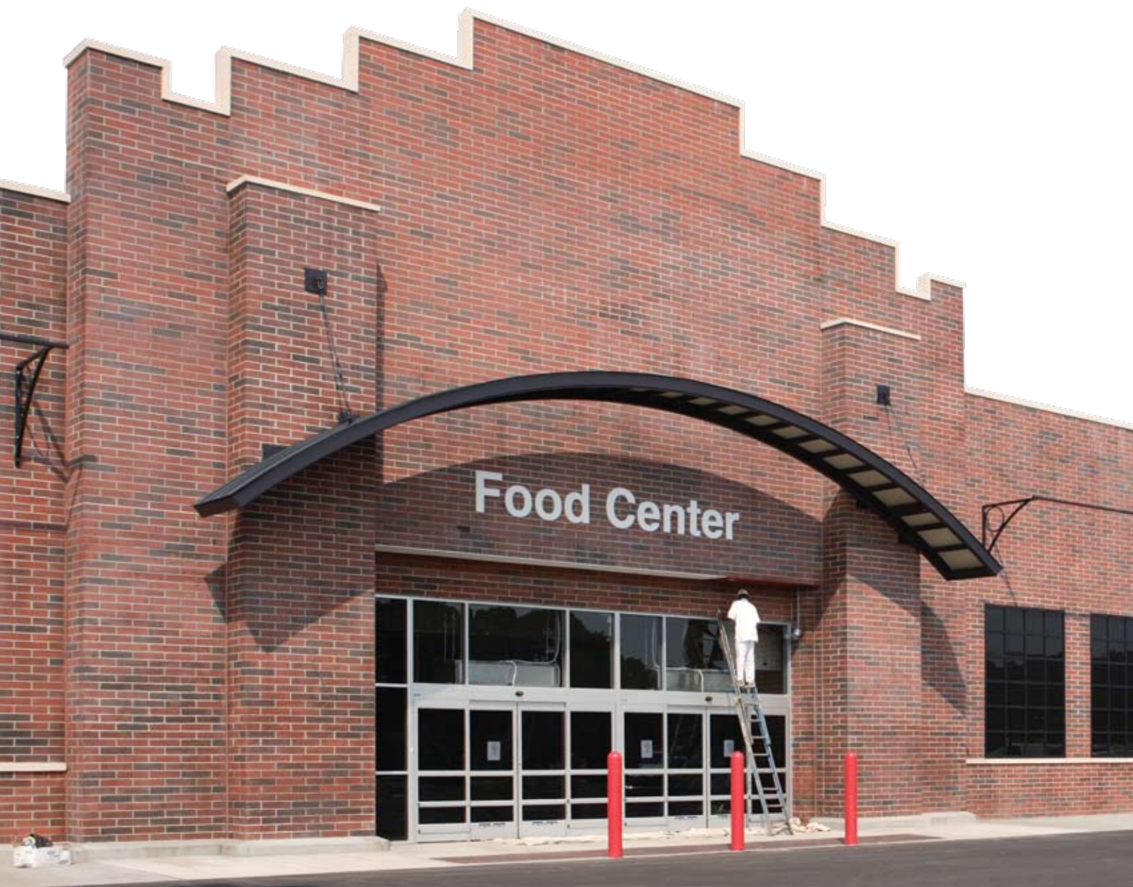
The new Eastwood Village, anchored by a Super Wal-Mart, features a single wythe of architectural half-high units. Some out parcels (right) feature a similar design.
